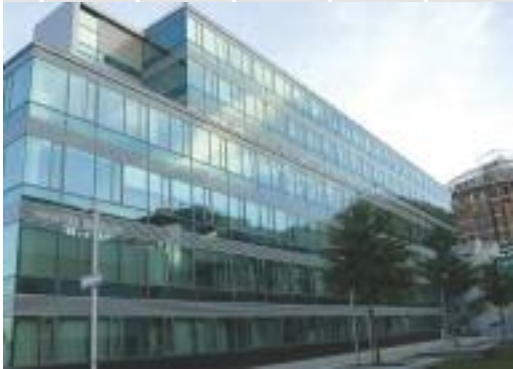
Office Campus Gasometer
